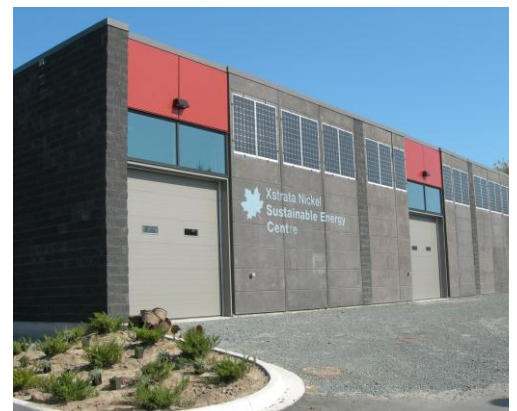
Xstrata Nickel Sustainable Energy Centre With @Source-Energy System
